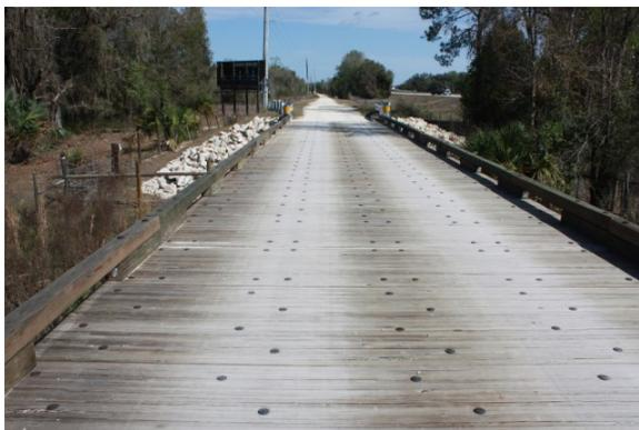
In addition to maintaining a one-lane bridge typical section and using timber as a construction material, the new bridge eschewed the use of barrier wall. In this case, the old bridge had been in place for nearly 50 years without any recorded incidents where an errant vehicle drove off the bridge. As a mix between CSS and Practical Design, the design team decided to replace the existing timber curb in-kind on the new structure. This approach not only saved money on barrier wall construction,
