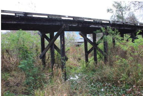
Standard FDOT bridge design would have replaced the existing bridge with a new concrete and steel structure. In addition, full implementation of FDOT roadway standards would have required two 12-foot lanes with 8-foot outside shoulders. Barrier walls would also have been required along the outside of the new structure to keep errant vehicles from falling off the bridge.
